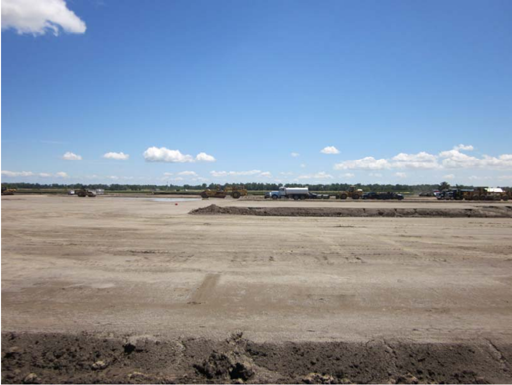
Photo 3: Final grading work at the compressor station site.
