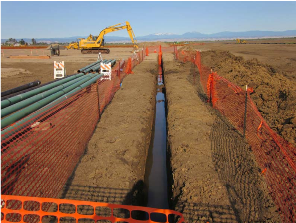
Photo 2: Gas line 172 trench at the remote well pad site.
