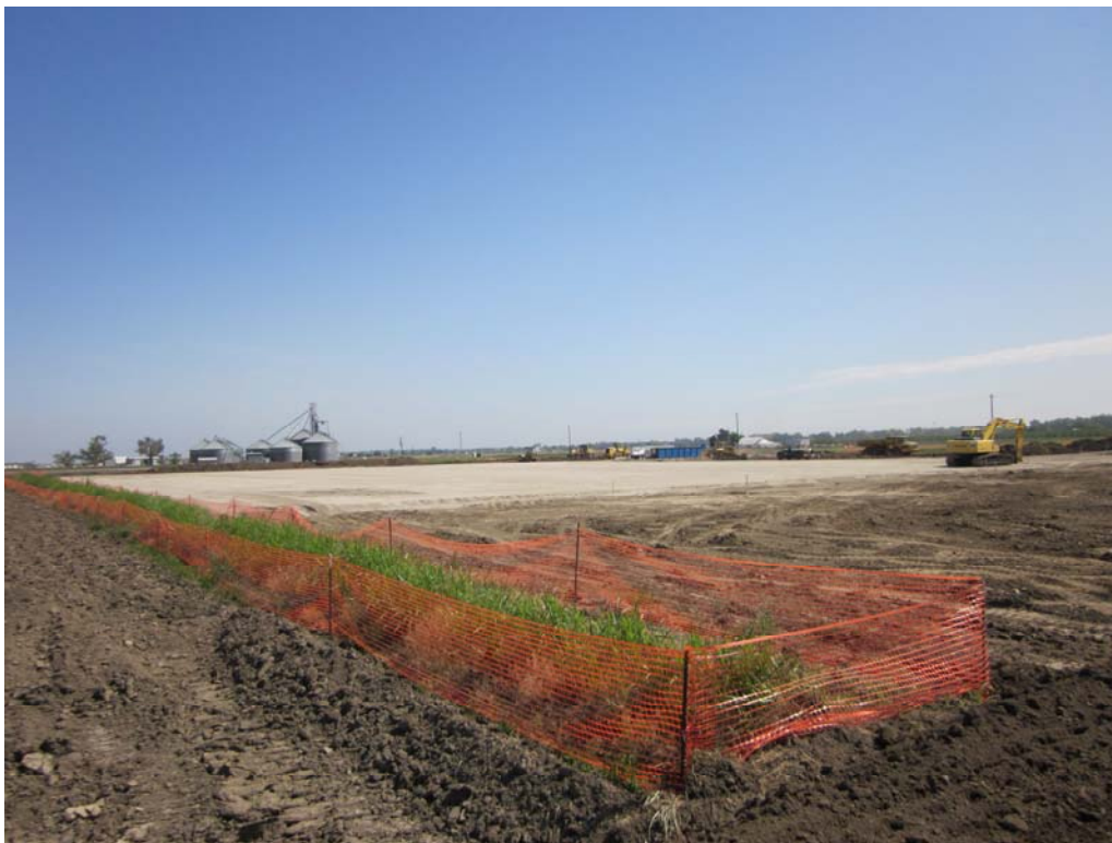
Photo 5: Exclusion fencing is placed around sensitive resource areas to minimize the potential for impacts outside of approved work areas.
