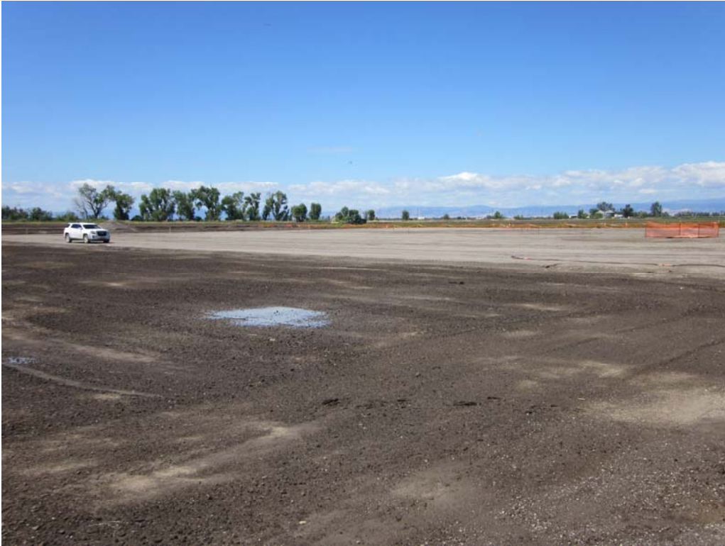
Photo 1: Final grading completed at the remote well pad site.
