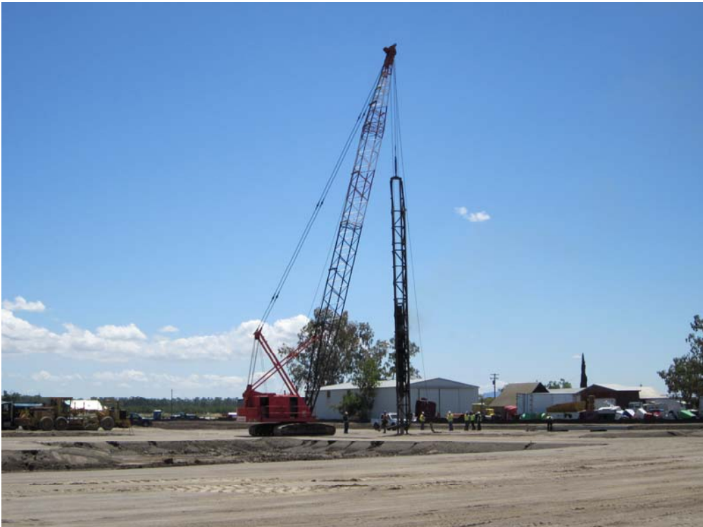
Photo 4: Driving of piles at the compressor station site.
